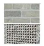
Wienerberger Forum Smoked Branco brick for the main exterior walls with the same bricks in a hit and miss design to be used for screens to the north and south elevations of terraces. Windows will be a dark grey aluminium framed casements, the main roof
